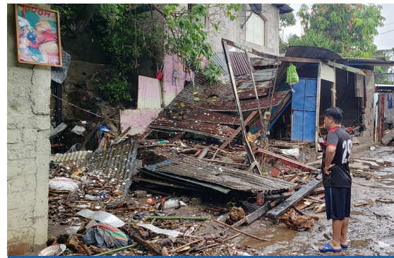
House demolished by hurricane Amanda, 6.20.
