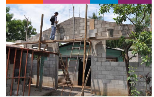
Work progresses on church façade in Agua Santa, Sonsonate, 6.15.
